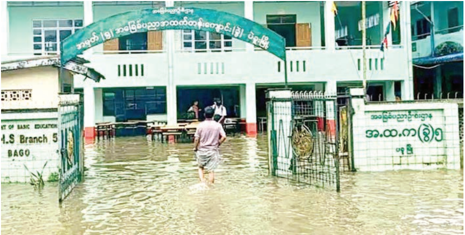
Floodwaters are entering some schools due to the rising Bago River.
