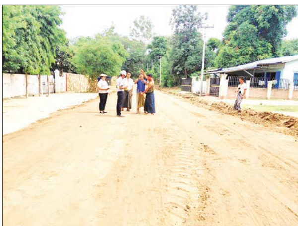
Officials oversee the road construction project in Yenangyoung Township on 2 September 2026.
