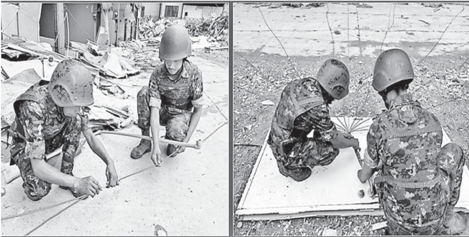
Personnel prepare to detonate a 17-storey illegal building used in online scams/gambling in Shwe Kokko Area, Myawady District in Kayin State.
