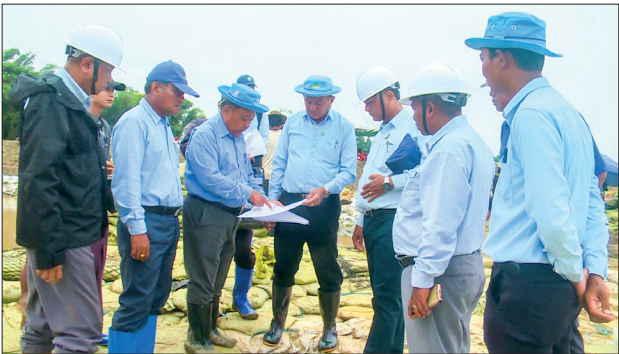
Officials inspect preparations to block water inflow in Hinthada Township.
