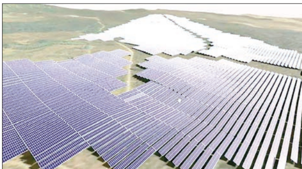
Solar panels gleam on a mountainside as Bhutan expands its renewable energy infrastructure. PHOTO: LINKEDIN
