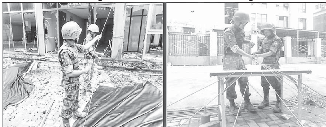
Personnel prepare to detonate a nine-storey illegal building used for online scams/gambling in Shwe Kokko Area in Myawady District in Kayin State.
