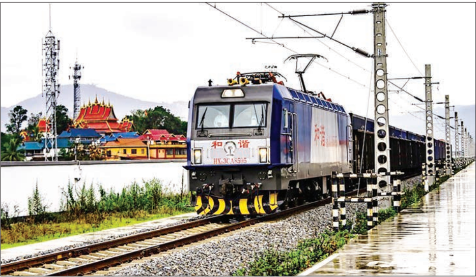
A freight train is to enter the China-Laos Railway’s Friendship Tunnel connecting Mohan in southwest China’s Yunnan Province and Boten in northern Laos, 24 November 2022. PHOTO: XINHUA/FILE
