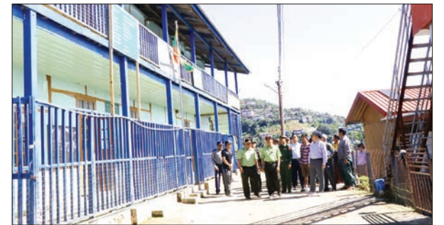
Deputy Minister Maj-Gen Kyaw Swa Oo inspects repair works in Chin State yesterday.
