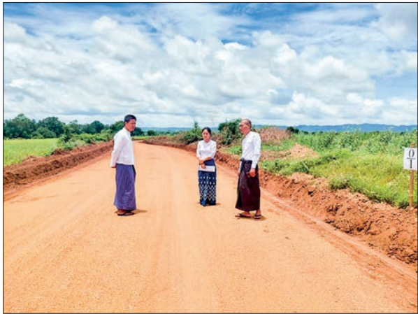
Officials inspect progress of paving laterite road in Minhla Township on 25 July.
