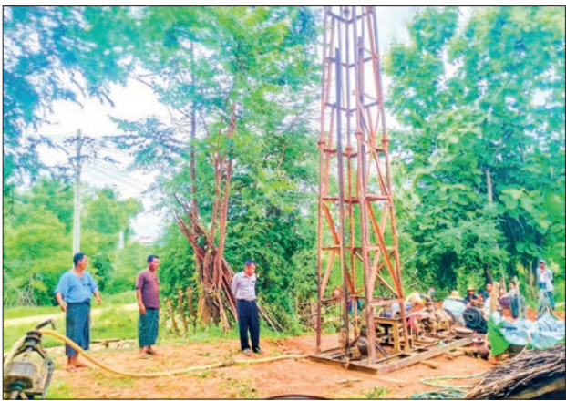
This photo shows a tube-well sinking rig at the water supply works in Sinbaungwe Township.
