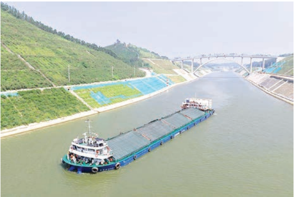
An aerial drone photo taken on 12 August 2026 shows a trial vessel driving past a bridge for animals over the Pinglu Canal in south China's Guangxi Zhuang Autonomous Region. PHOTO: XINHUA
