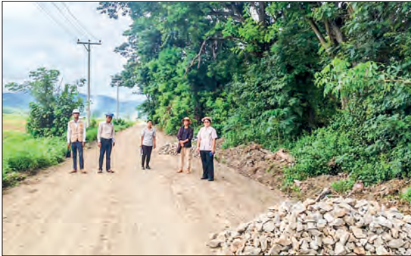
Officials oversee the ongoing asphalt paving work on inter-village roads in Mawkmai Township.
