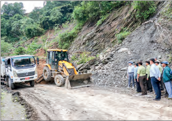
Deputy Minister Maj-Gen Kyaw Swa Oo and officials inspect road repairs and reconstruction efforts in Chin State.
