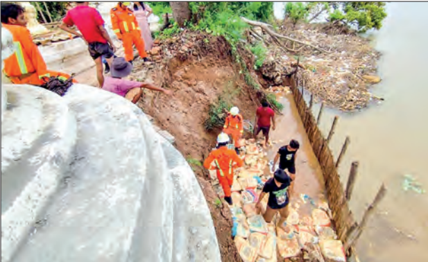
Relevant organizations and fire brigades are carrying out emergency protection and maintenance work to prevent the collapse of the retaining wall.
