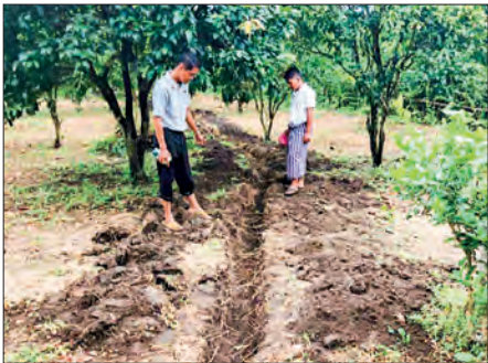
Officials inspect the construction of the irrigation pipeline in Machanbaw Township.
