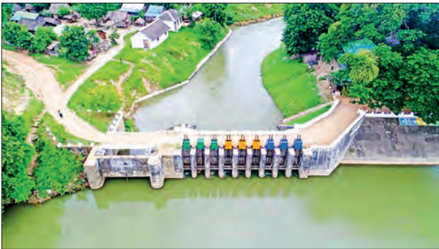
Photo shows Aingma Diversion Weir which distributes irrigation water to monsoon paddy fields in Minbu (Saku) Township. PHOTO: MAUNG MAUNG (MINBU)
