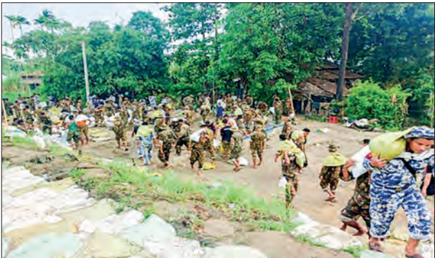
Volunteers participate in repairing damaged Nyaungdonkyun embankment.
