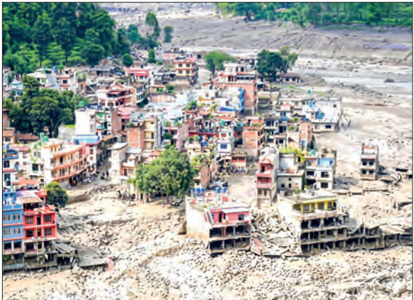
Principal successfully evacuates nine hundred students before school structure collapses. PHOTO: INSTAGRAM
