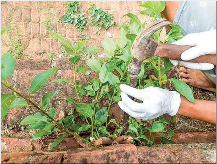
Cleaning the trees growing on the pagoda platforms with chemical solutions.
