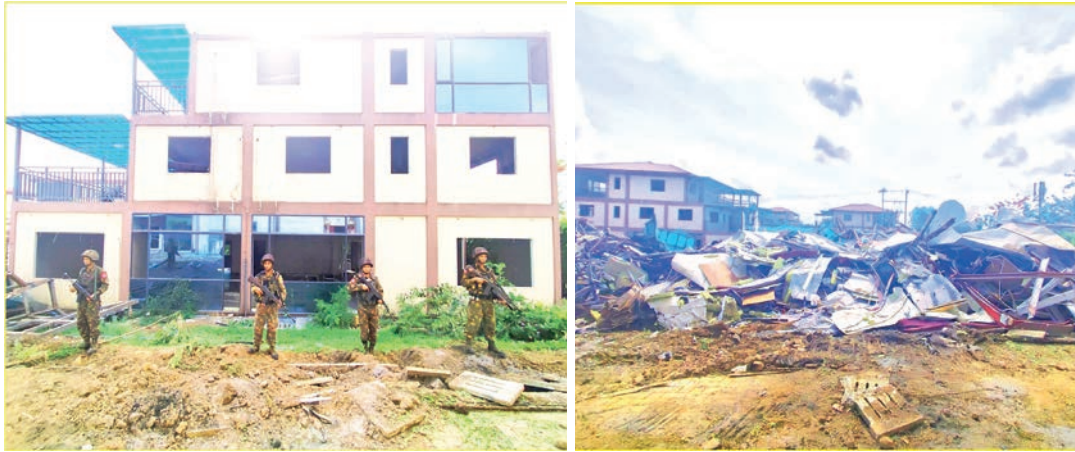
Images reveal the update before and after the demolition.
