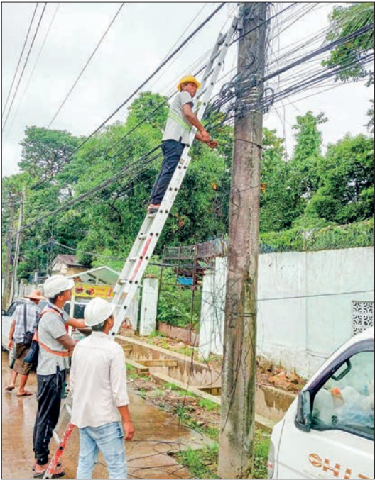
Illegally installed Wi-Fi cables and dangerous telecommunications cables are being removed. PHOTO: CHIT SAUNG - YESC
