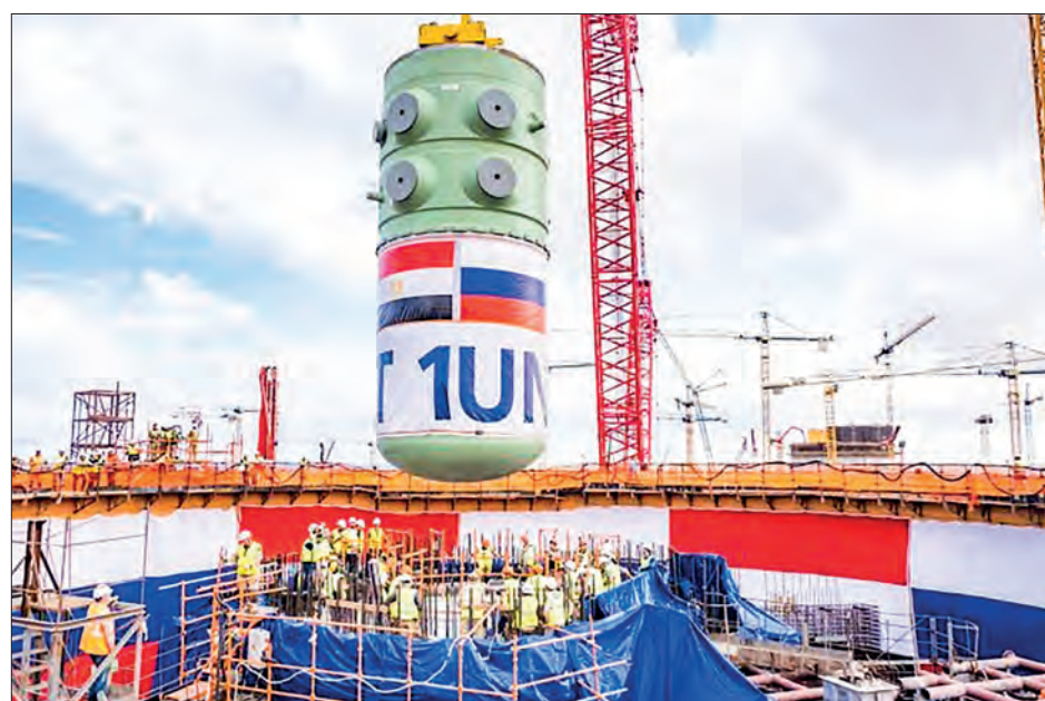
This image shows the installation of a 330-tonne reactor pressure vessel for Unit 1 at the El Dabaa Nuclear Power Plant in Egypt. PHOTO: ROSATOM
