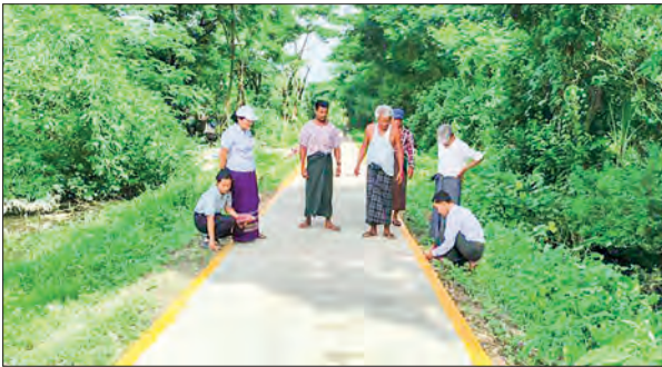
This image features the completed Mya Sein Yaung concrete road project in Khayan Township.
