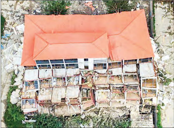
Image displays the update after the demolition of a nine-storey structure.
