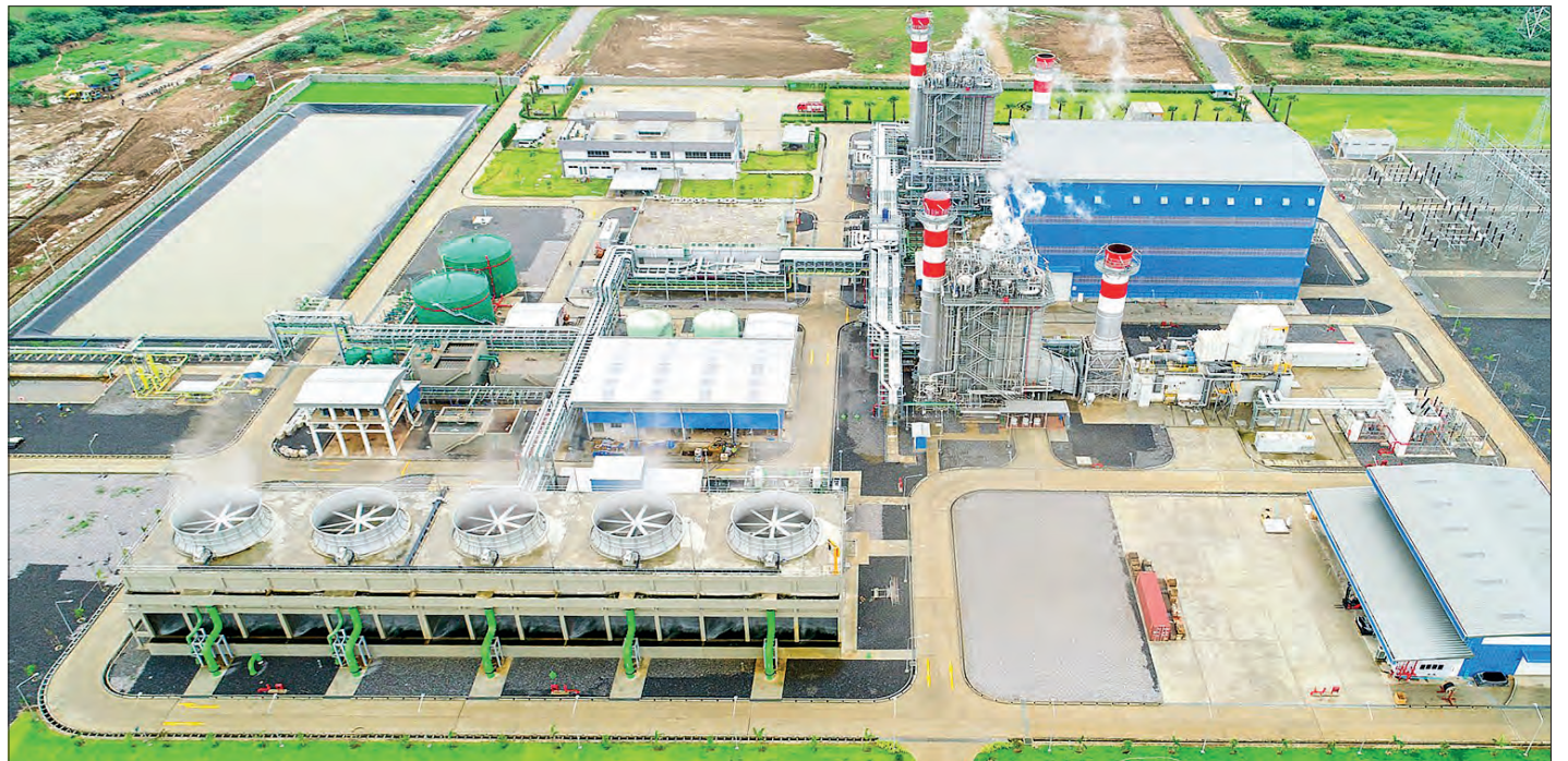
A power plant generating electricity in Myanmar.
