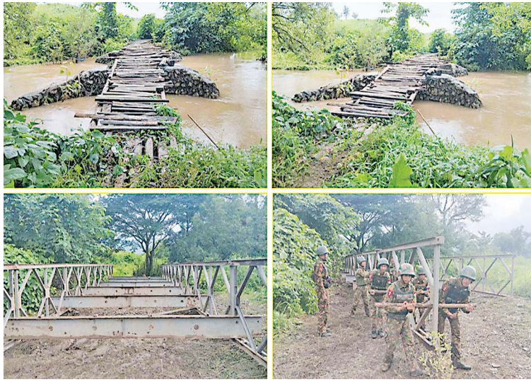
Ongoing repair work on the Kyunkhunnapin Bridge destroyed by terrorist insurgents.
