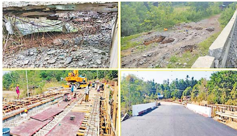
Completion of repairs to Five-Pole Bridge destroyed by terrorist insurgents.
