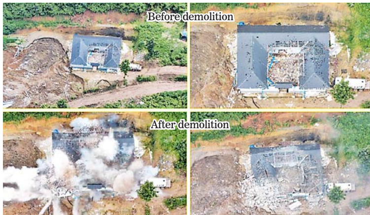
Demolition of illegal buildings used for online scam and gambling operations in the Kyauk Khet Area.
