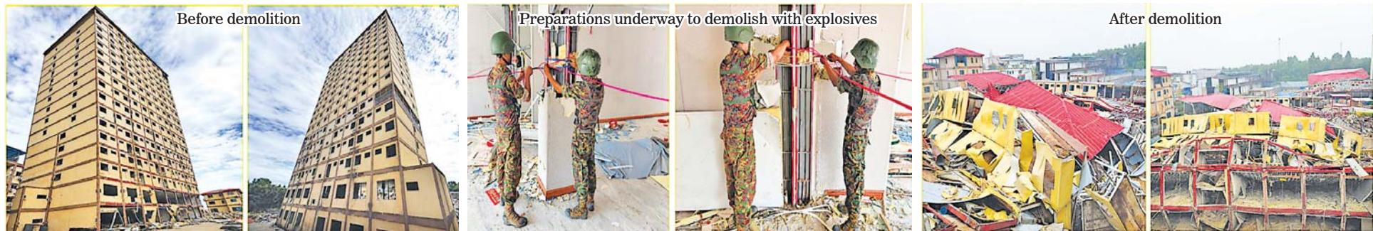
An illegal 17-storey building used for online scam and gambling operations in the Shwe Kokko Area, Myawady District, Kayin State.
