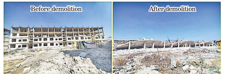
Demolition of an illegal four-storey residential building in the KK Park Area.
