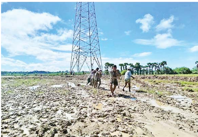
Electricians and employees are repairing a transmission tower.
