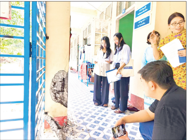
The Myanmar Earthquake Committee officials inspecting the structural integrity of the building.
