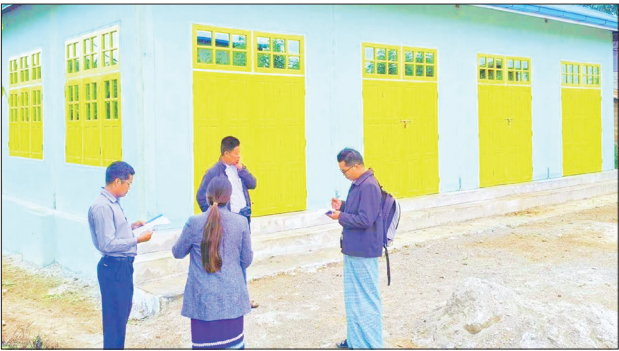
Officials from the Department of Rural Development inspect the completion of a multi-purpose hall in Kalaw Township.
